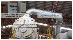
Oxygen Sensor for Monitering Hot Water Boiler
